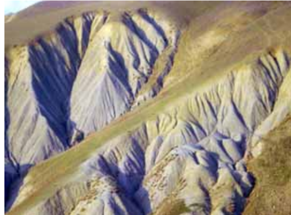
Fig. 4. The watershed upstream erosion of the Boughezoul dam; photo: B. Remini
