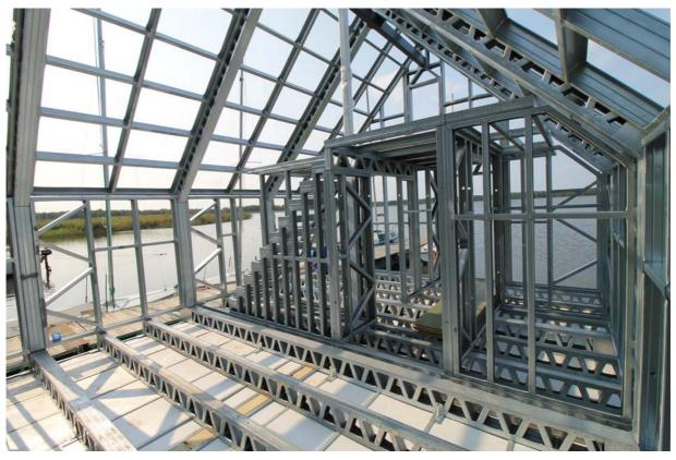
Fig. 5. Scottsdale Construction System structure raised on the steel and styrofoam platform before insulating; source: own elaboration
