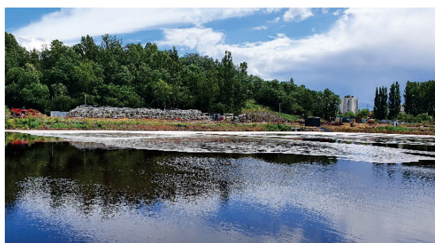
Photo 2. The Kalina pond – view on the reclaimed area with the visible effect of action of the installed aeration nozzle system (phot.: K. Starzec)
