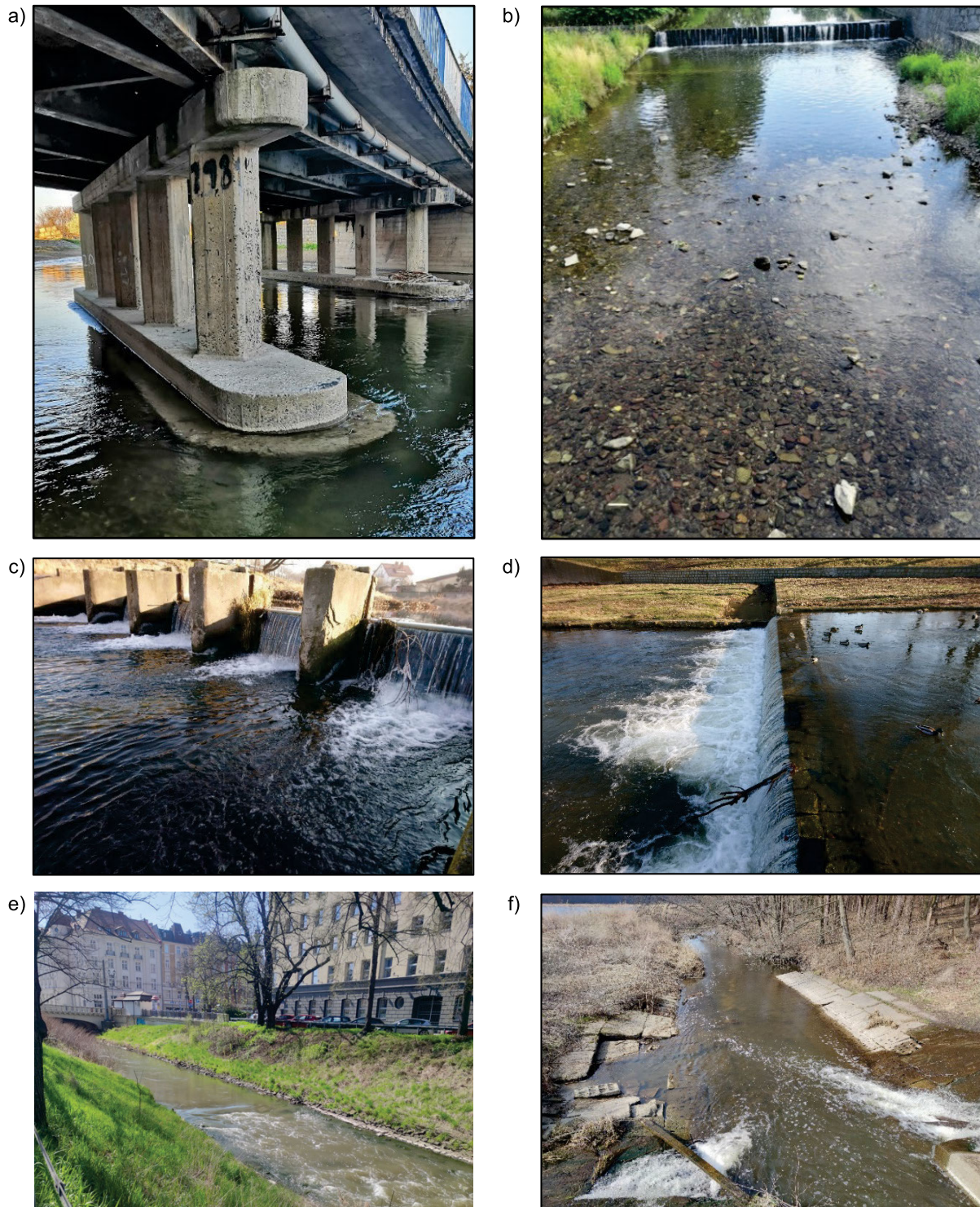
Photo 1. River valley morphological elements included in the River Habitat Survey method: a) bridge piers (the Bystrzyca River), b) visible bottom granulation (the Bystrzyca River), c) concrete weir (the Pilawa River), d) hydraulic jump visible downstream the stone weir (the Bystrzyca River), e) transition from smooth to turbulent forms of water movement (the Kłodnica River), f) devastated bed and riparian concrete reinforcement (the Czarna River) (phot.: M. Kiraga)
