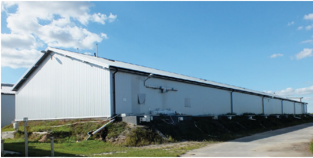
Photo 2. 1.6 MWe biogas plant (ProBioGas linear technology) in Miedzyrzec Podlaski with separated hydrolysis and the possibility of biohydrogen production (phot.: J. Dach)
